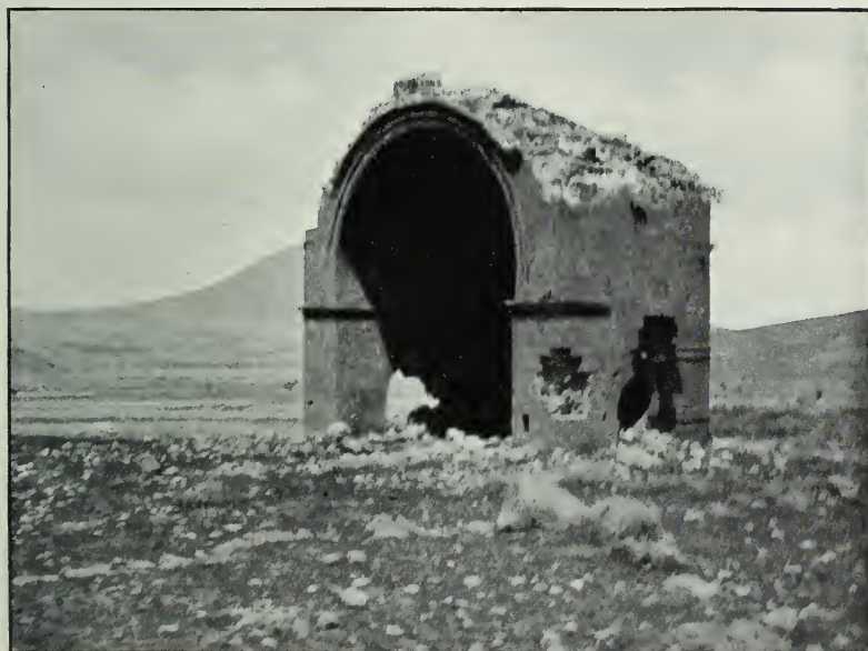
FIG. 49.—No. 7, exedra, from S.-W.
